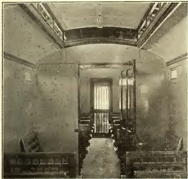
Montreal Prison Car—Interior of Car, Showing Part of Both Compartments
