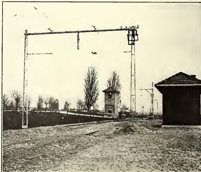
Vienna-Pressburg Single-Phase Line—View of Typical Steel Pole and Bridge Catenary Construction
