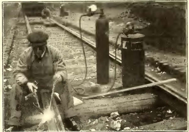
Making a Joint by Means of Oxy-Acetylene Weld
