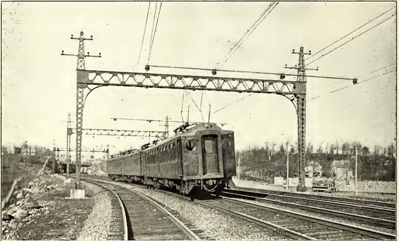
Westchester Equipment—Typical Three-Car Train
