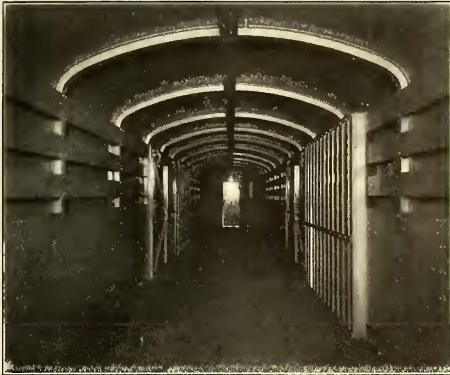
Interior, Showing Unit Carline and Post Construction
