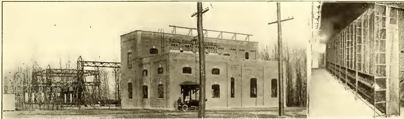
Substations—Indoor-Outdoor Substation at Agawam—Framework for Bus Structure
