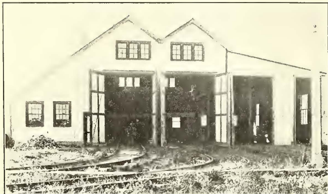
Edmonton City Maintenance—Temporary Car Sheds, South Side, Edmonton
