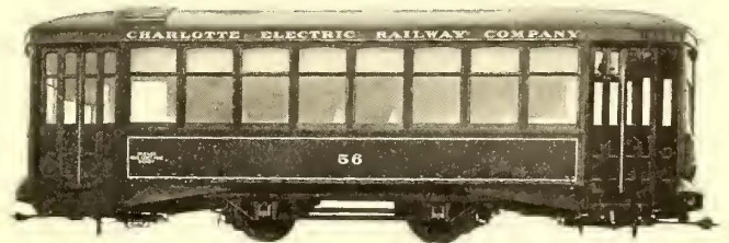
Charlotte Electric Railway—Single-Truck Vestibule Car
