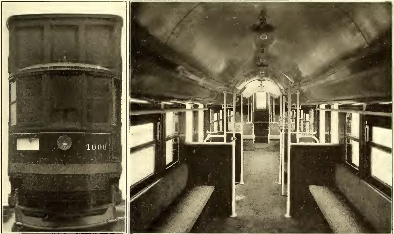
Columbus Double-Deck Car—Views of Front of Car, Showing Motorman's Cab and Fender Arrangements, and of Lower Deck Interior
