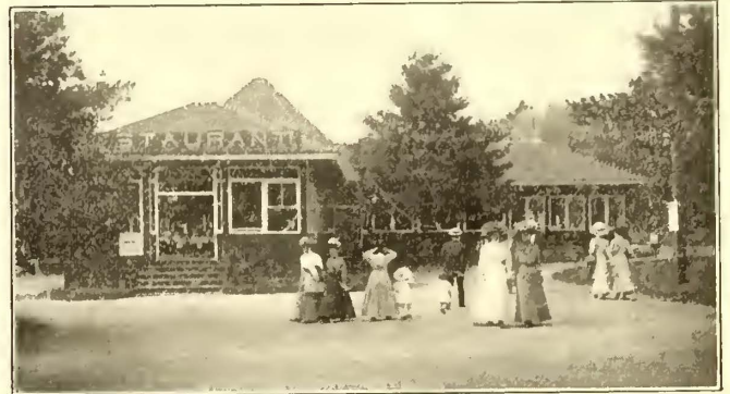
Canobie Lake Park—Large Restaurant; Roof Outlined with Incandescent Lamps
