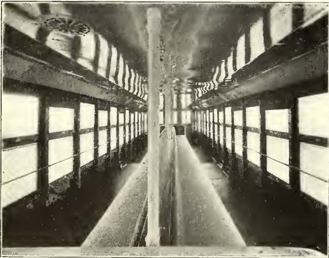
Columbus Double-Deck Car—Interior of Upper Deck
