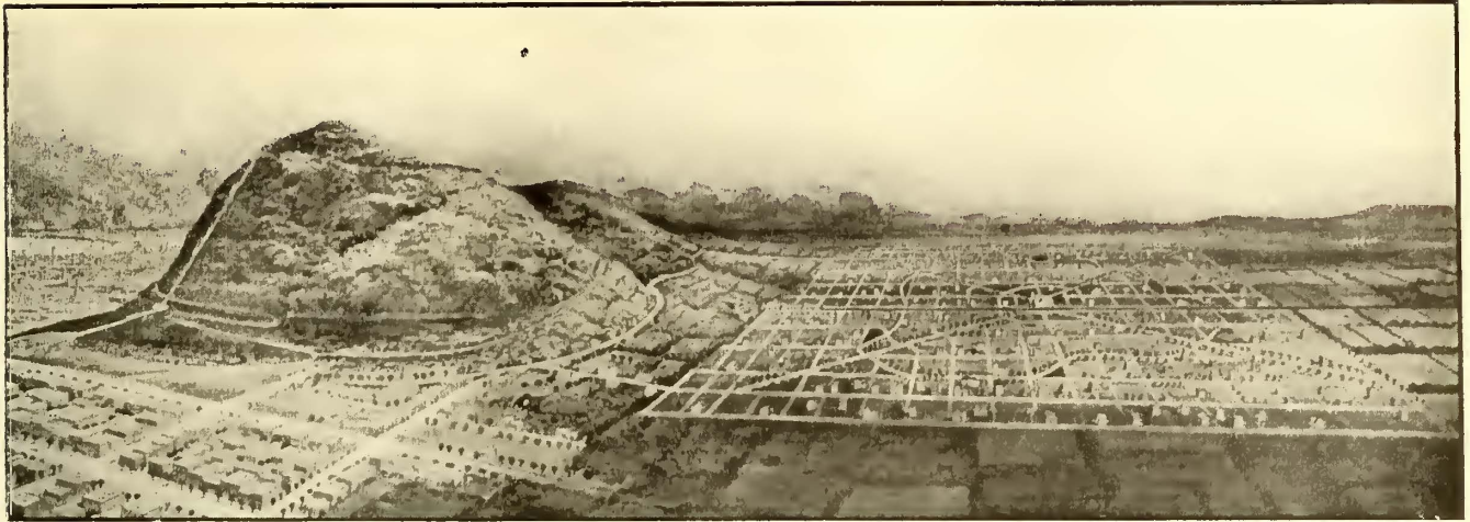
Fig. 3—Montreal Tunnel—Bird's-Eye View Showing How the Tunnel Will Develop the Territory on the Far Side of Montreal
