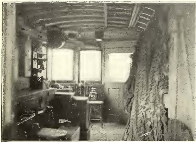
Toledo Derrick Tower Car—Interior View
