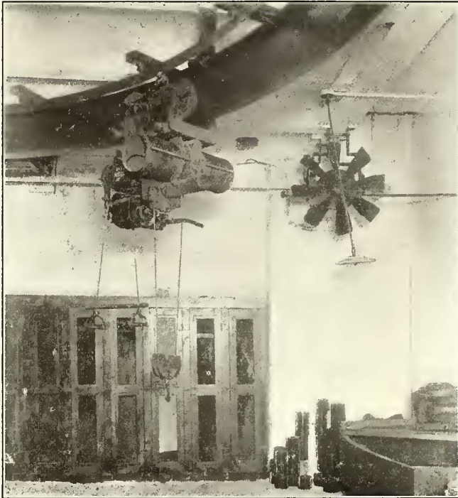
Third Avenue Motor Shop—Telpher Hoist, Ventilating Fan and Lockers.
