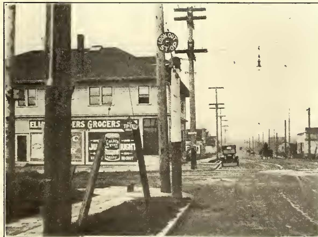
"Wigwag" Signal to Give Visible and Audible Warnings at Perilous Street Intersections
