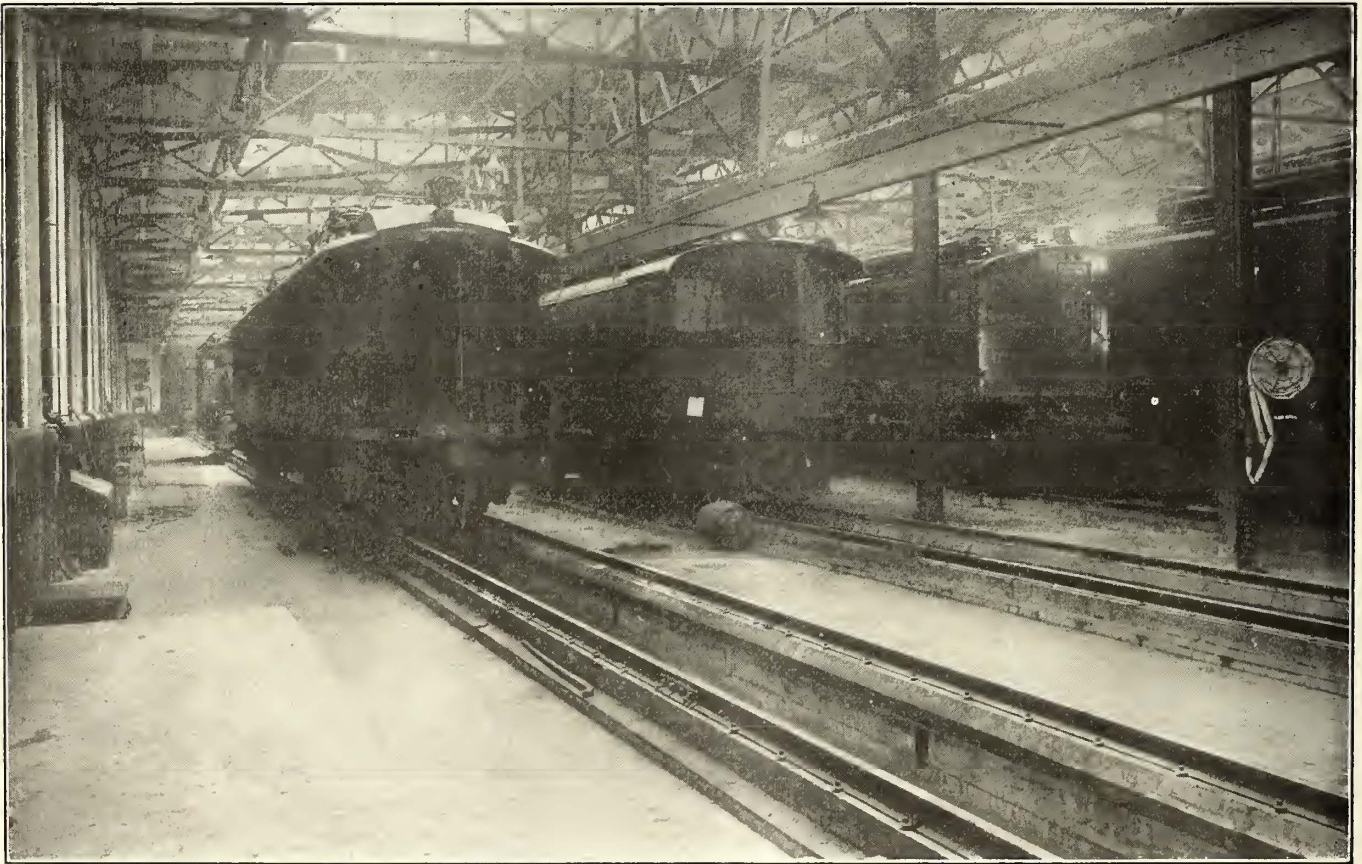
New Haven Shops—Interior of Inspection Shed
