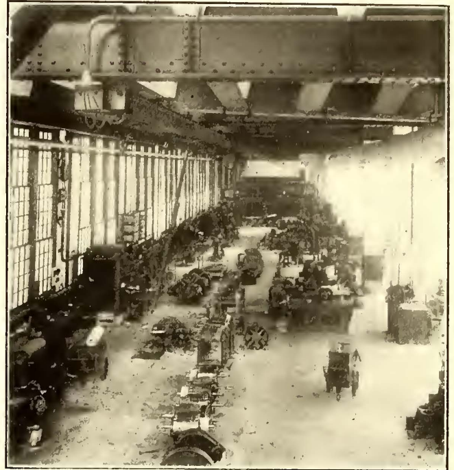
New Haven Shops—East End of Light Tool Bay
