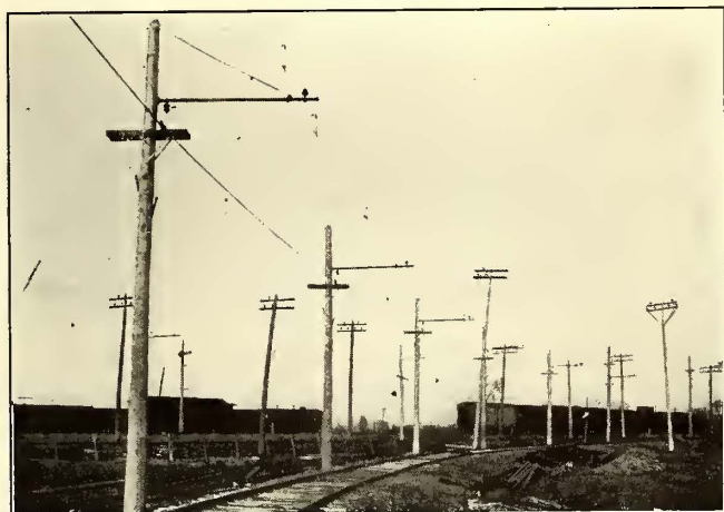
Montreal & Southern Counties Railway—Catenary Work on Curve
