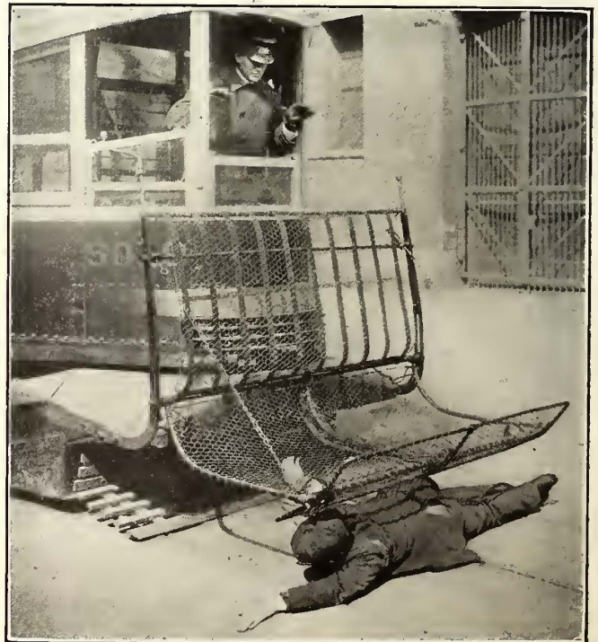
Safety First in New York—Action of Fender Gate in Dropping Wheelguard
