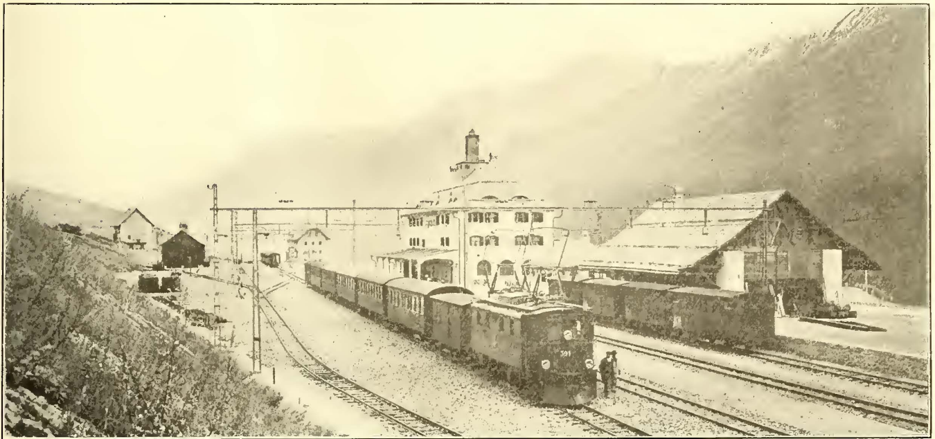
Rhaetian Railway—Light Steel Catenary Bridges at Schuls-Tarasp Station
