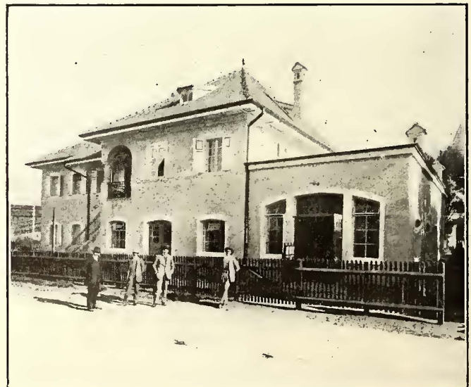
Ueberetsch Railway—Combined Substation and Residence at Etschwerke
