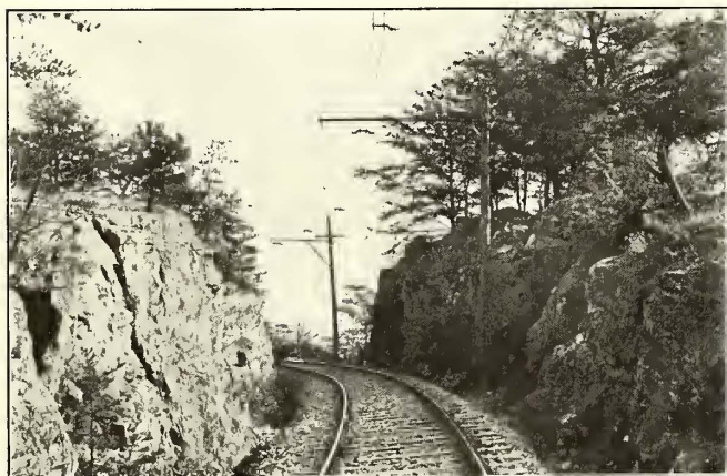
Lookout Mountain—A Typical Rock Cut on the New Right-of-Way
