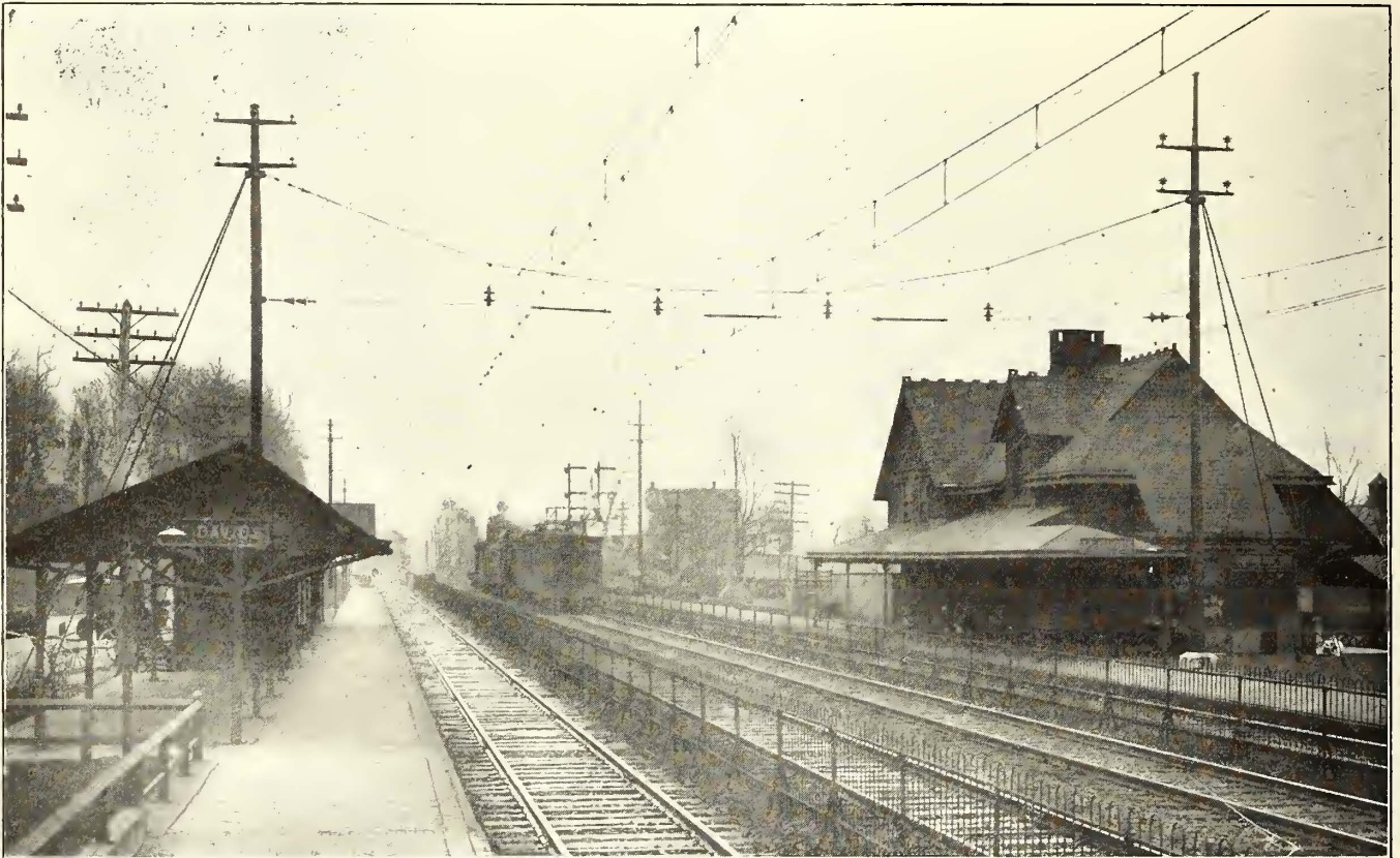
Philadelphia Electrification—View of Experimental Installation on the Main Line Showing Preferred Type of Construction Over Left-Hand Track—Test Cars in Background
