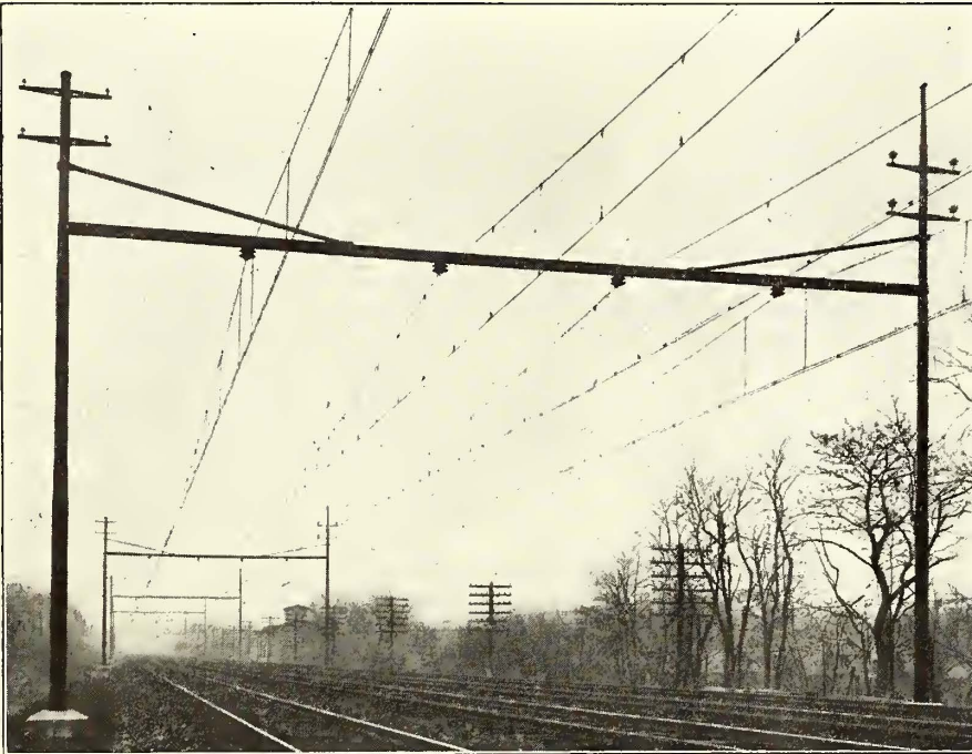
Philadelphia Electrification—Views of an Experimental Form of Catenary Bridge. The Cross-Catenary Type of Supporting Structure Has Been Found to Be Superior to This and Will Be Used for the Permanent Installation
