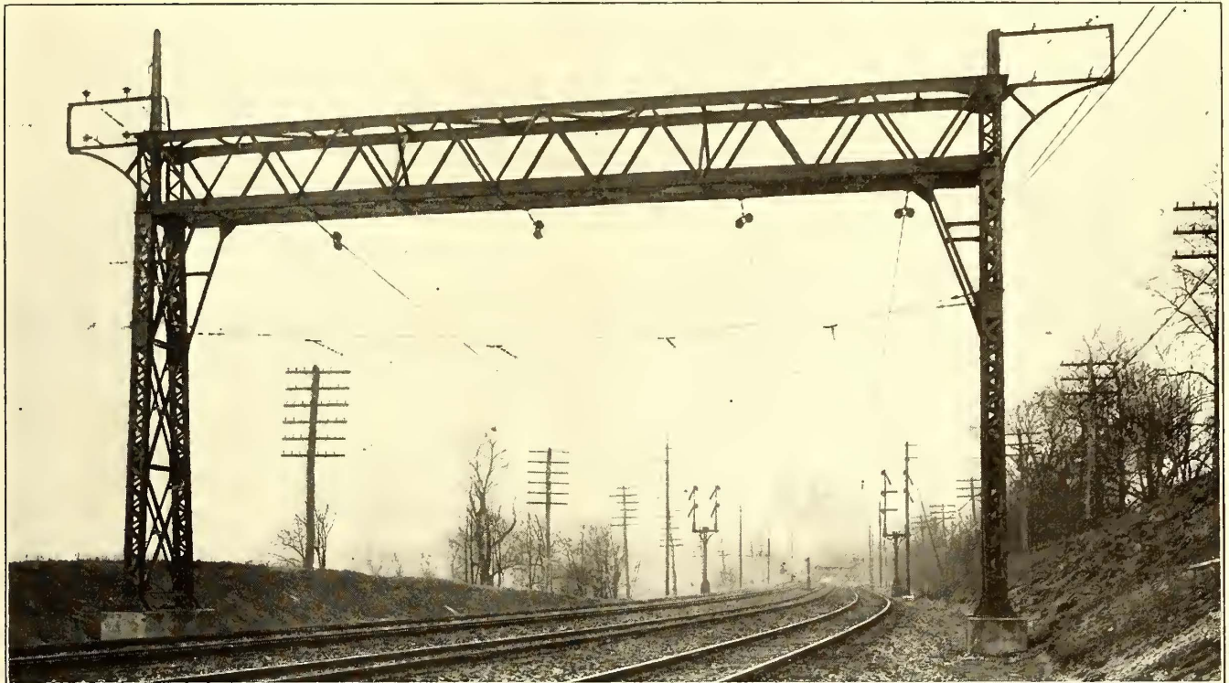
Philadelphia Electrification—View at End of Experimental Section of Track Showing Construction of Anchor Bridges Which Will Be Installed at Half-Mile Intervals
