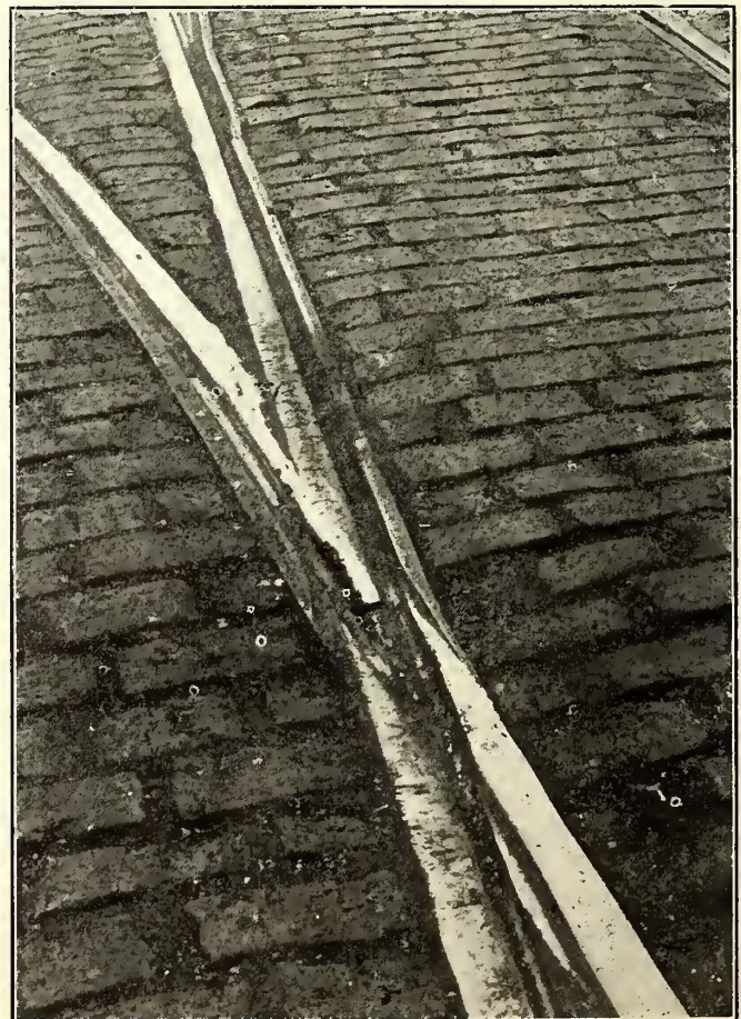
Chicago Special Work—Fig. 16—Showing Extreme Case of Crumbling in Manganese Frog, Installed April, 1909; Traffic, 176 Wheels Per Hour
