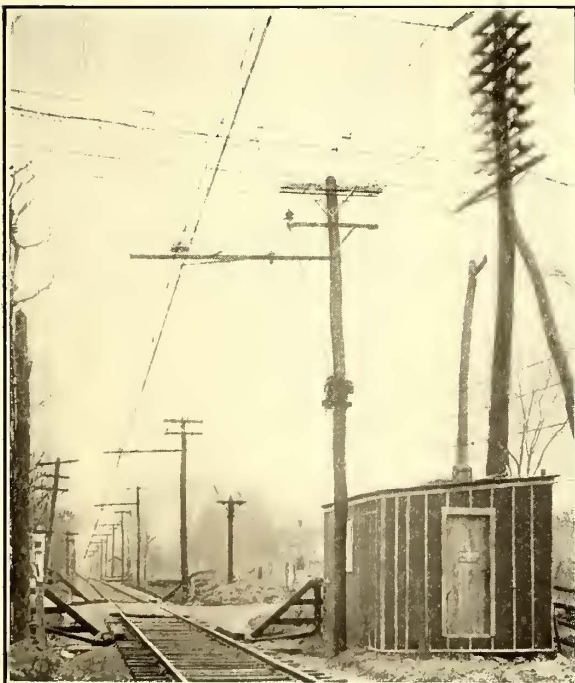
New Haven Electrification—Fig. 19—Instrument House on New Canaan Branch
