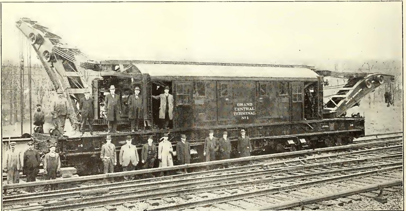
Electric Wrecking Crane—General View of Crane with One Boom Swung 90 Deg. Off Center
