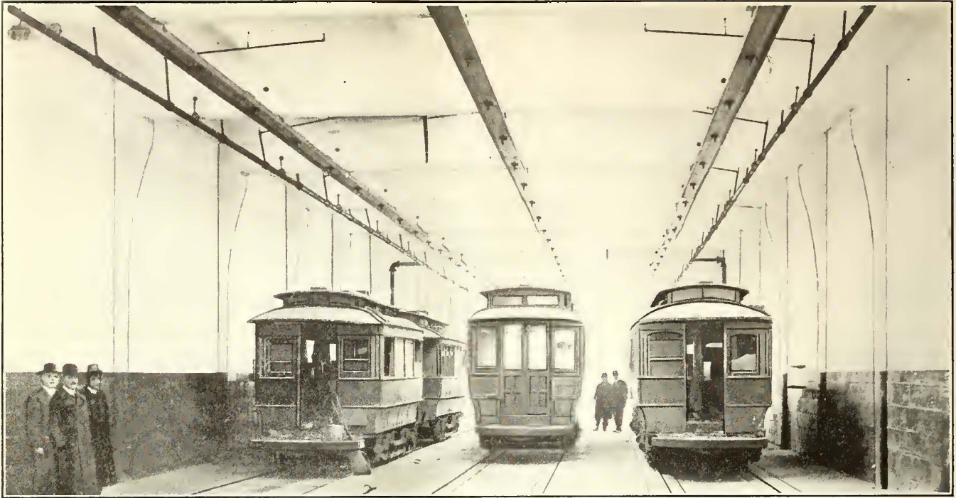
Philadelphia Sprinkler Test—Fig. 1—Conditions Before Start of Fire, Showing Layout of Sprinklers with Test Car on Middle Track
