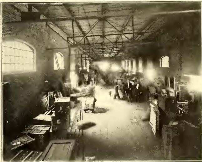
Detroit Freight and Express—Interior of Inbound Warehouse
