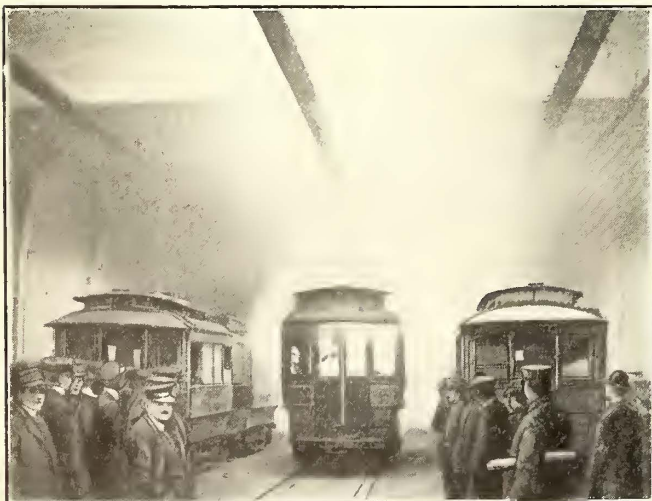
Philadelphia Sprinkler Test—Fig. 2—Start of Fire After Glass was Broken to Give Draft
