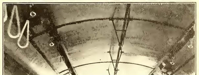
Albany Cars—Ceiling Detail, Showing Truss Plank from Which the Lamps and Straps Are Carried
