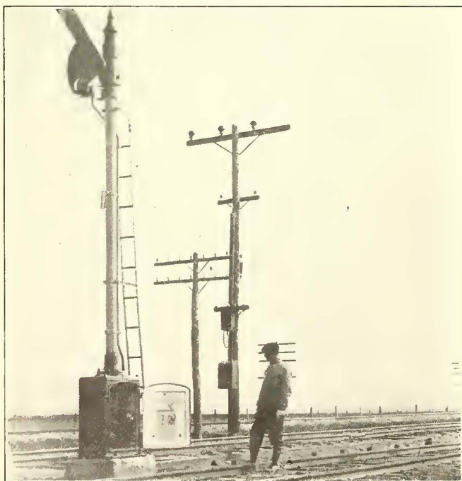
Illinois Signal Maintenance—Signal Operating Mechanism Exposed for Repairs
