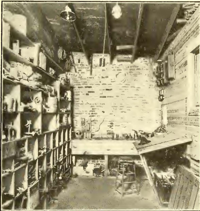
Illinois Signal Maintenance—Interior of Telephone Repairman's Shop
