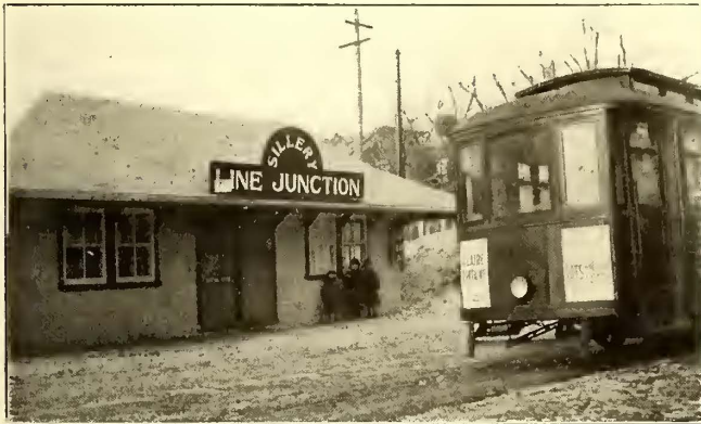
Quebec Traffic Development—Passenger Station of Wood Faced with Tin
