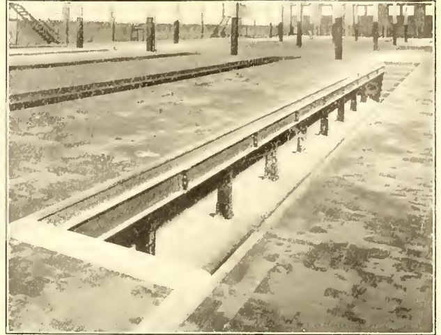
Detroit United Machine Shop—View of Repair Pit in Truck Shop
