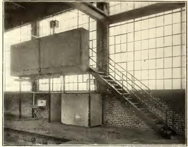
Detroit United Machine Shop—View Showing Typical Toilet Balcony
