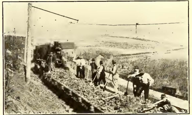
Seattle Municipal Railway—Work of Rehabilitation of Highland Park & Lake Burien Railway
