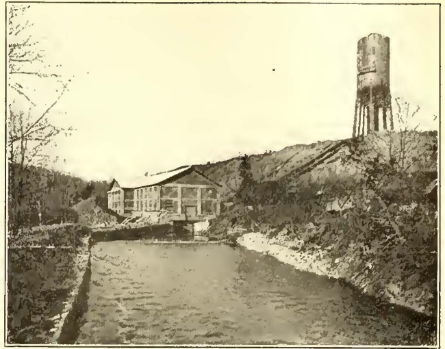
Salmon River Power Development—Power House, Surge Tank and Tailrace
