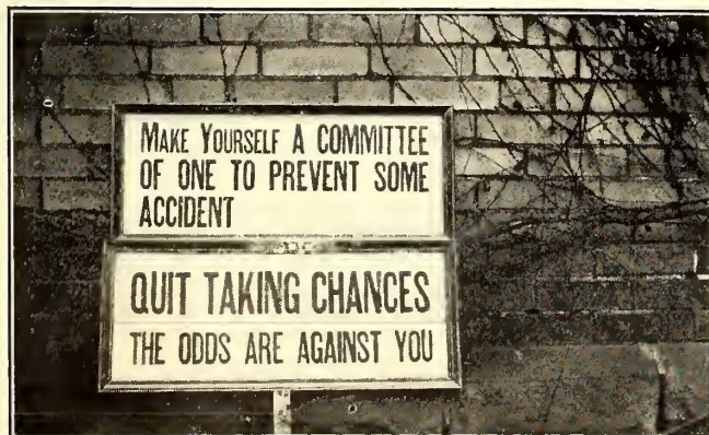
"Safety First" in a Small City—Fig. 2—Signs at Carhouses and Shops
