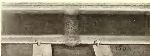
Finished Thermit Fully Welded Insert Rail Joint
