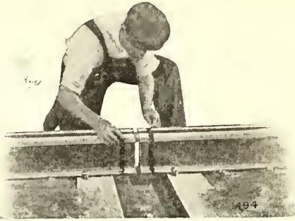
Applying Asbestos and Molasses Strips to Rails Previous to Adjusting Mold
