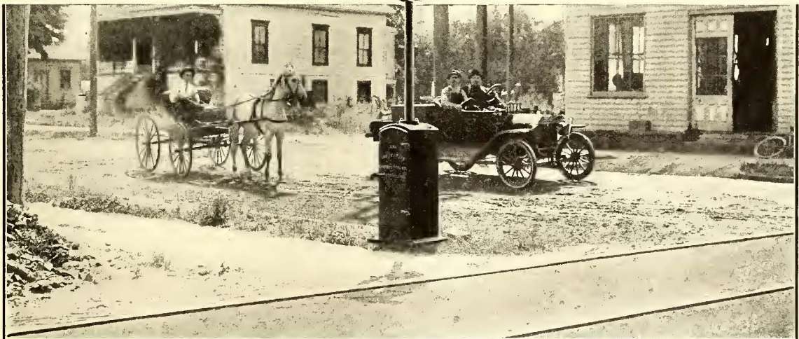
Typical Crossing Protection on the Petaluma & Santa Rosa Ry., Santa Rosa, Cal.
