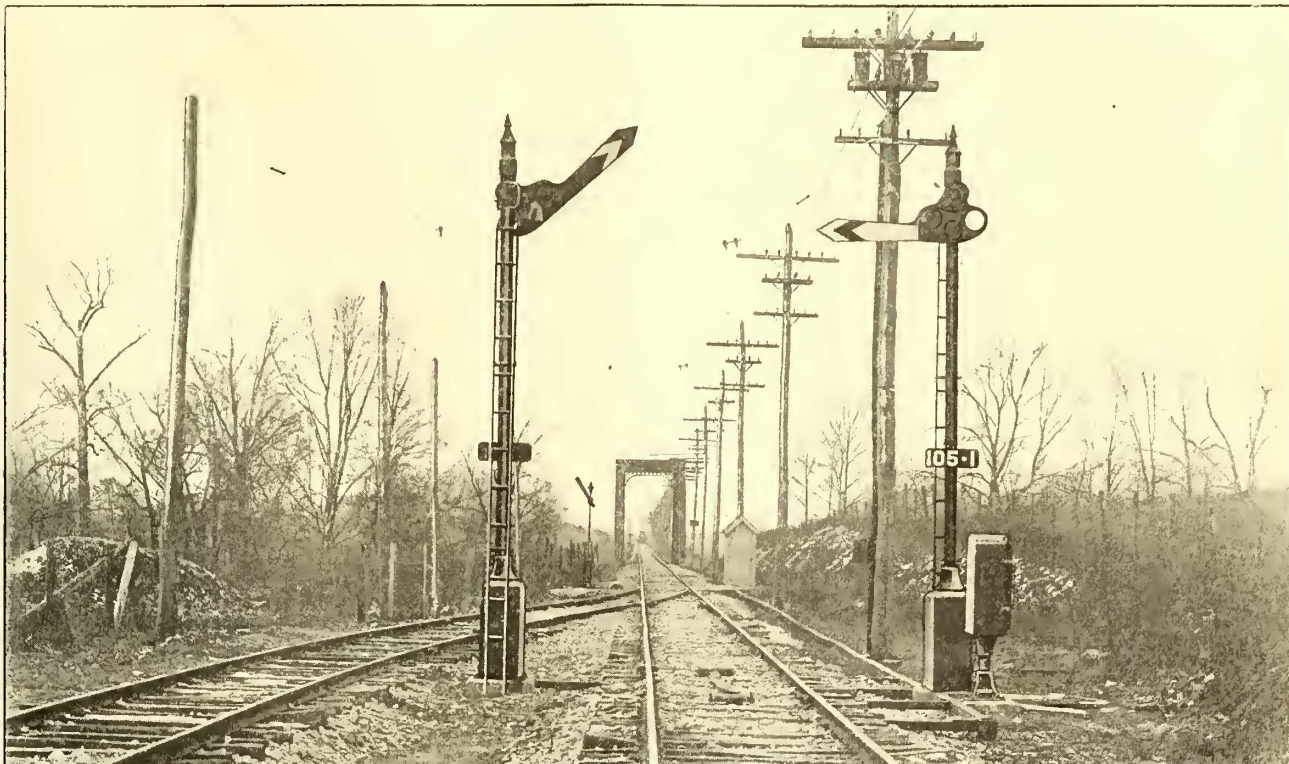
Style "B" A.C. Automatic Block Signals at Turn-out on Louisville & Northern Railway & Lighting Co. The TDB System.
