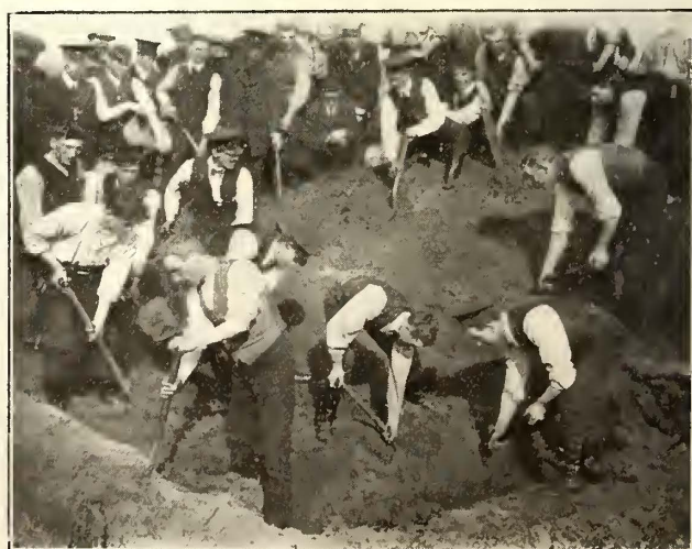
GLASGOW'S RAILWAY SOLDIERS—A LESSON IN CUT AND COVER TRENCH CONSTRUCTION
