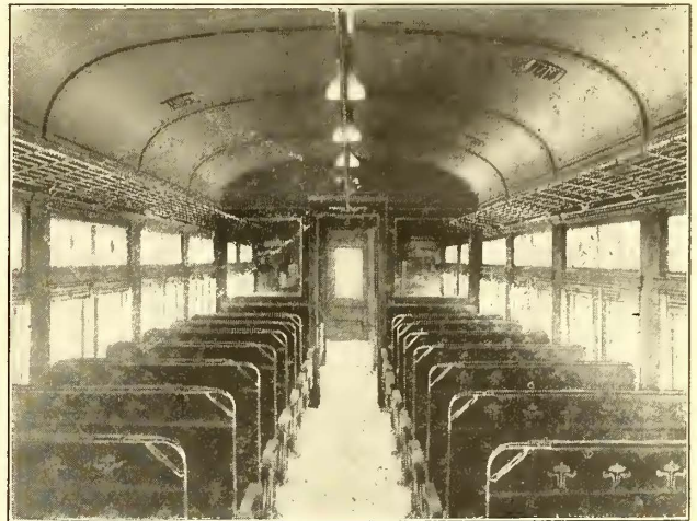
SALT LAKE & UTAH RAILROAD—INTERIOR VIEW, SHOWING LOCATION OF VENTILATORS AND LAMPS
