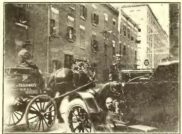
SAFETY FIRST—CAUTION SIGNS ON AUTOMOBILES AND WAGONS AT MONTREAL
