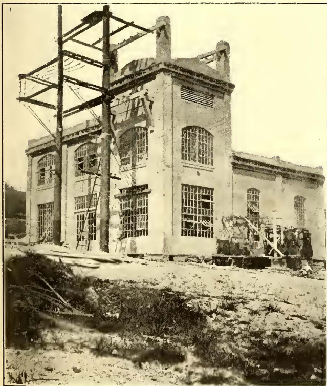
SEATTLE MUNICIPAL RAILWAY—EXTERIOR VIEW OF SUBSTATION
