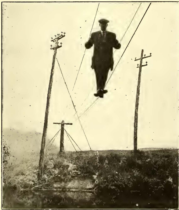
LINEMAN WALKING OVER CABLE TO SAVE A LONG WALK ON THE GROUND
