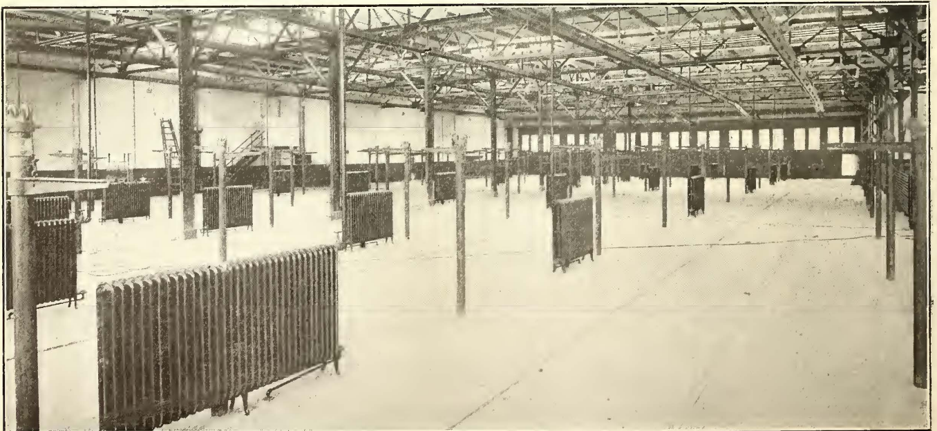
CLEVELAND SHOPS—INTERIOR VIEW OF PAINT SHOP
