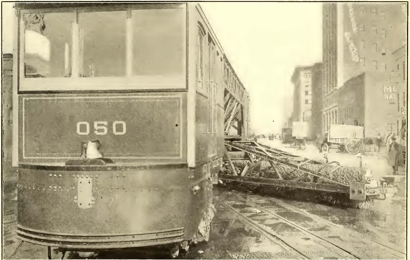
NEW YORK SNOW-SWEEPER—REAR VIEW SHOWING ARRANGEMENT OF WARNING LIGHTS AND BELL AT END OF BROOM
