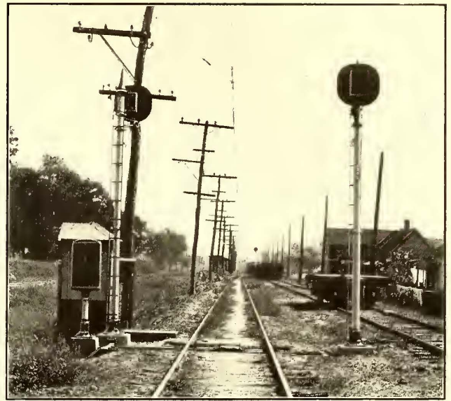
ILLINOIS TRACTION SIGNALS—VIEW OF SIGNALS AT TORRENCE SIDING ON THE DECATUR BELT LINE
