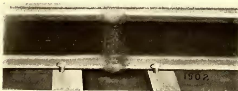
Finished Thermit Fully Welded Insert Rail-Joint
