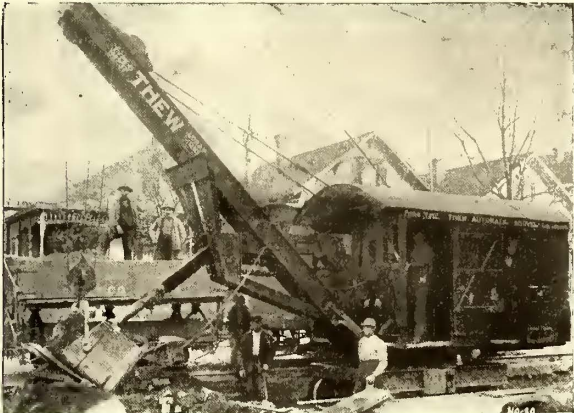
Thew Shovel making a shallow cut for track foundation, Indianapolis. Note pieces of concrete, rocks, etc.
