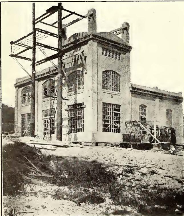
SEATTLE MUNICIPAL RAILWAY—EXTERIOR VIEW OF SUBSTATION
