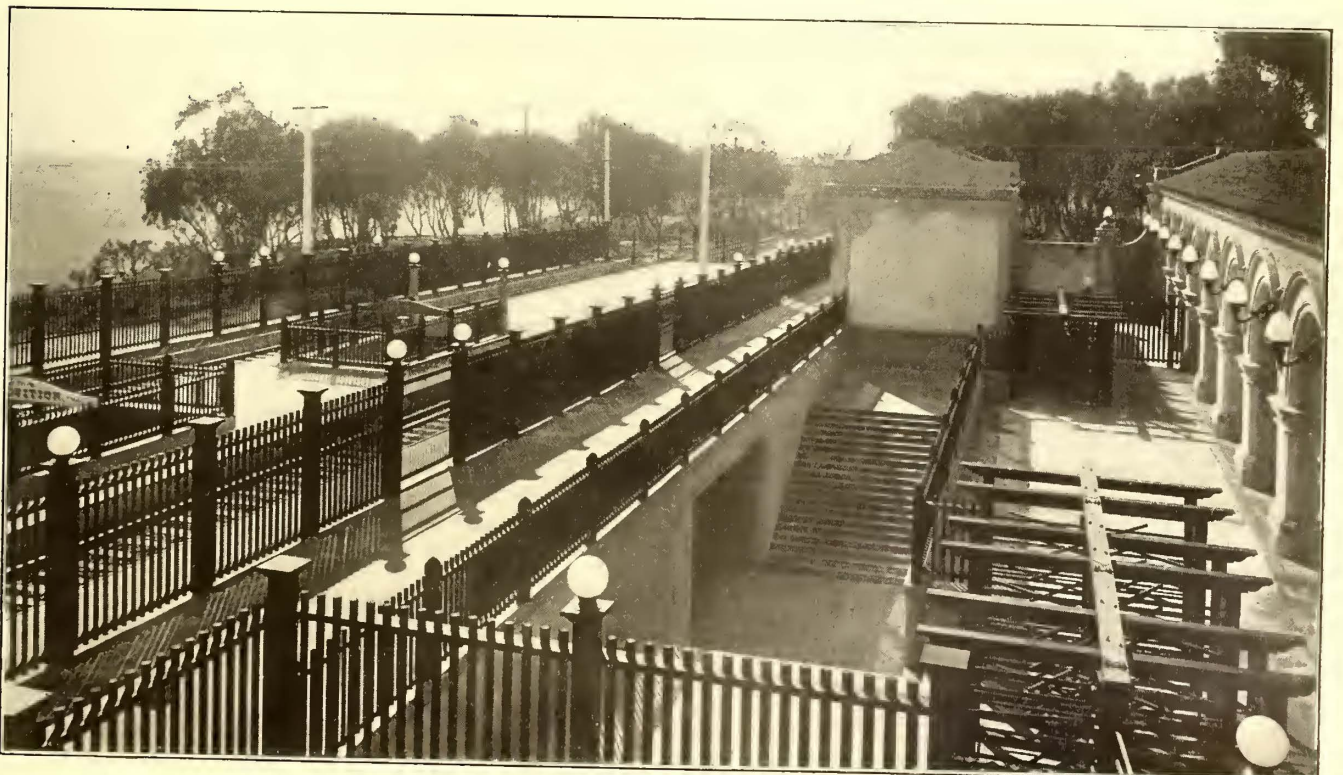
SAN DIEGO TERMINAL—GENERAL VIEW OF PLATFORMS
