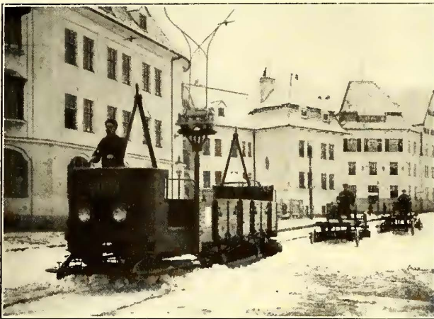
MOTOR CAR WITH PLOW FOR TRACK CLEANING AND WAGON TRAILERS FOR REMOVING SNOW BETWEEN RAILS AND CURB
