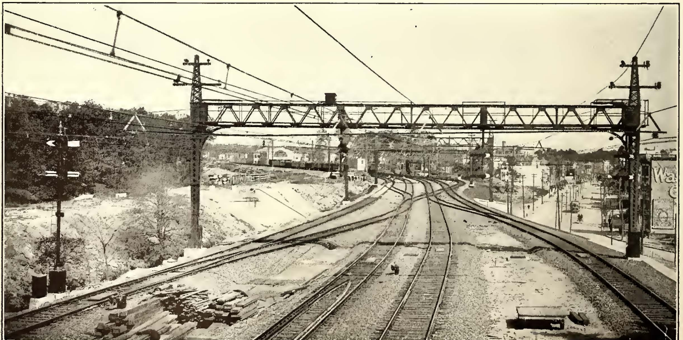
WESTCHESTER SIGNALS—CROSS-OVERS AND STORAGE YARD SIDING NORTH OF 180TH STREET INTERLOCKING PLANT
