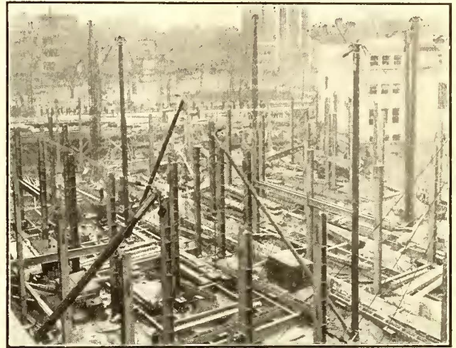
NEWARK TERMINAL—BIRD'S-EYE VIEW LOOKING NORTH-WEST, SHOWING STEEL COLUMNS
