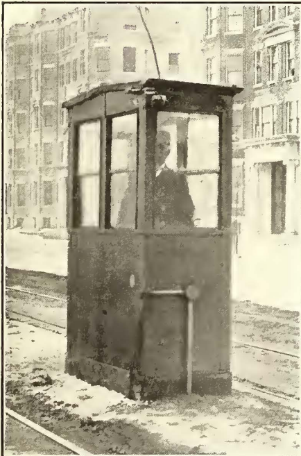
DISPATCHING SURFACE CARS AT BOSTON—DISPATCHER'S BOOTH; SIGNAL CONTROL INSTALLATION OVER TRACK
