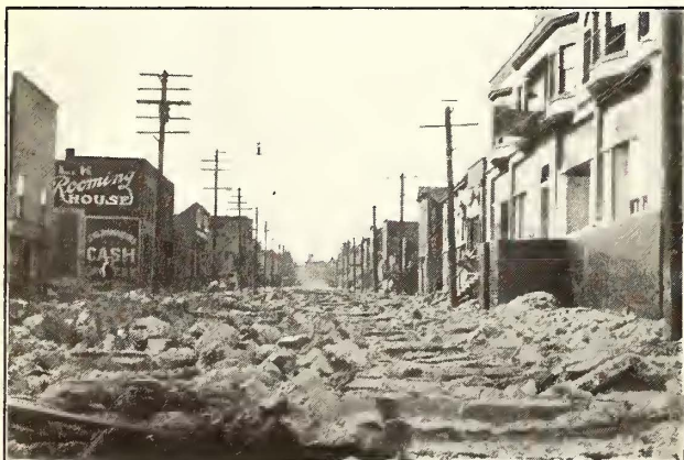
SEATTLE STREET GRADE—BALLARD AVENUE READY FOR HEAVY FILL
