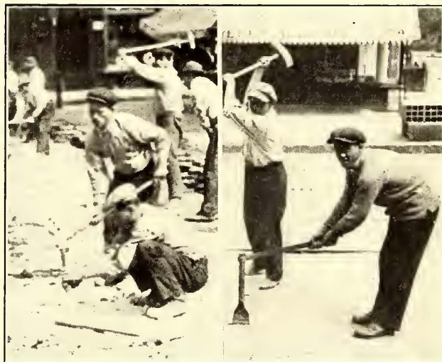
SAFETY-FIRST IN CUTTING CONCRETE PAVING FOUNDATION
