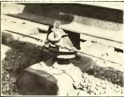
ATTACHING SIGNAL WIRES TO THIRD RAIL—FIGS. 1, 2 AND 3, SHOWING DIFFERENT ATTACHMENTS
