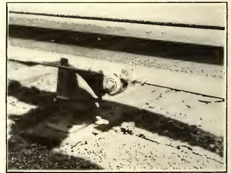
ATTACHING SIGNAL WIRES TO THIRD RAIL—FIGS. 1, 2 AND 3, SHOWING DIFFERENT ATTACHMENTS
