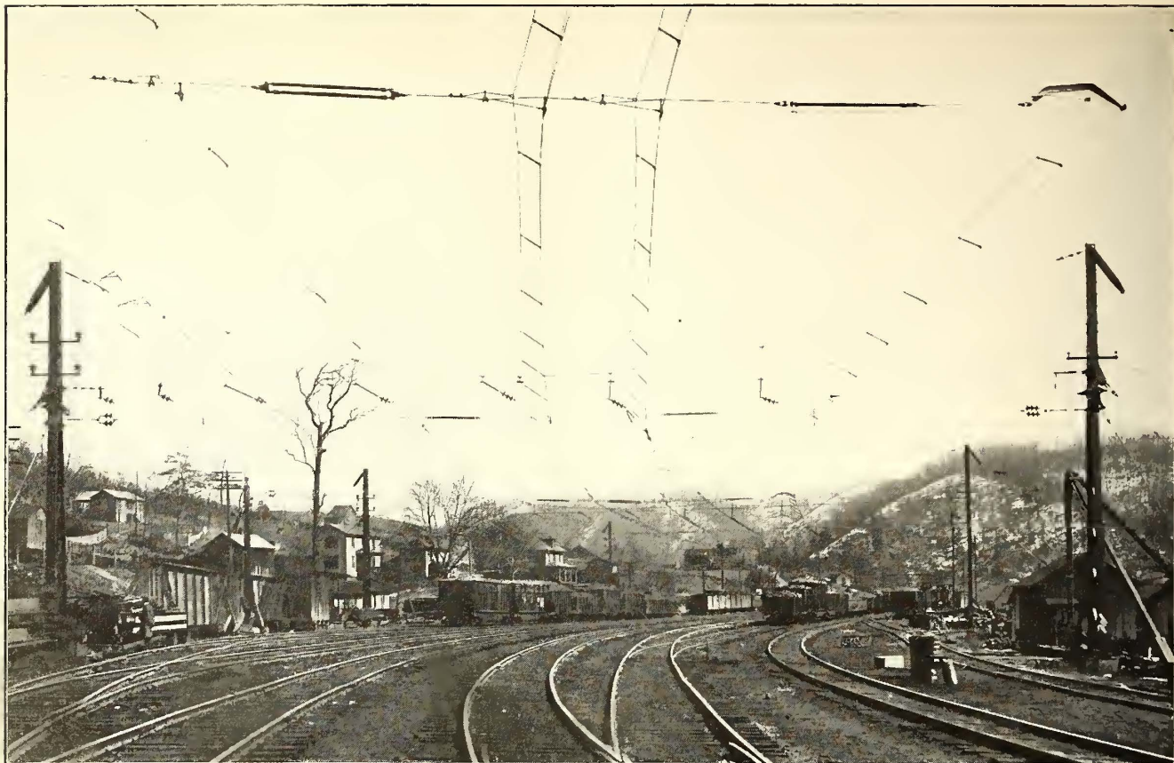
NORFOLK & WESTERN ELECTRIFICATION—CROSS CATENARY USED FOR YARD TRACKS
