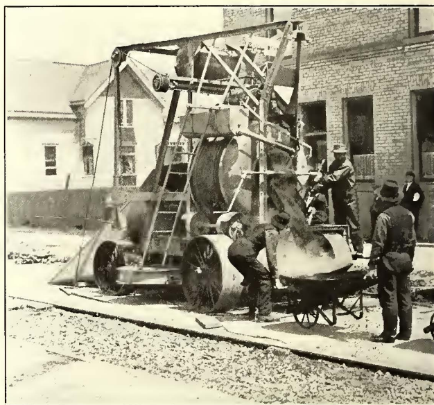
MILWAUKEE PAVING—DISCHARGING HOT REMIXED ASPHALT
