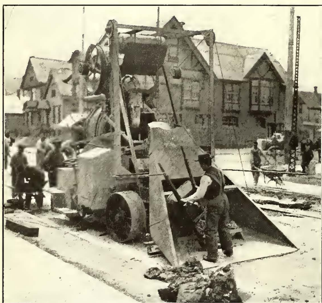
MILWAUKEE PAVING—LOADING OLD ASPHALT INTO HOT MIXER
