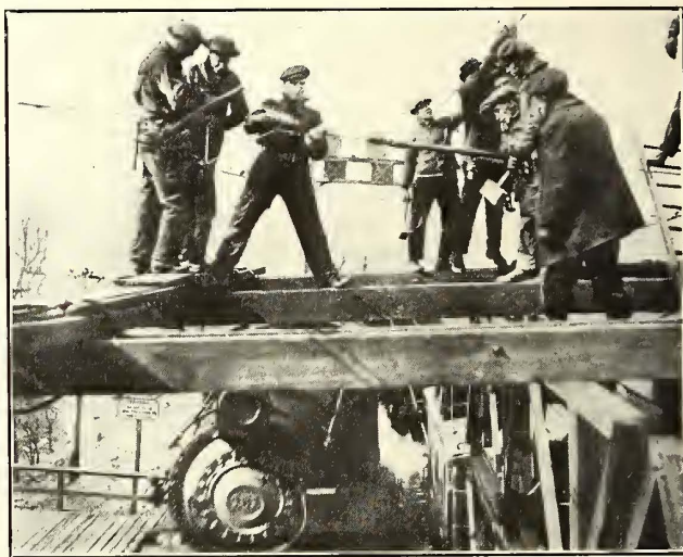
CONSTRUCTION GANG ON PHILADELPHIA-PAOLI ELECTRIFICATION STRINGING WIRES WITHOUT INTERRUPTING TRAFFIC
