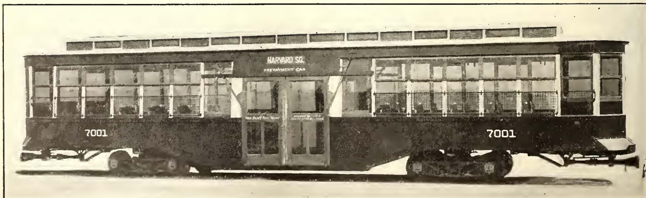
BOSTON CENTER-ENTRANCE TRAILER—EXTERIOR VIEW
