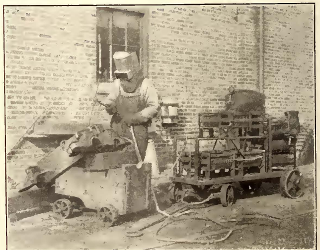
HAMPTON SHOPS—HOME-MADE WELDING OUTFIT IN USE ON A MOTOR SHELL
