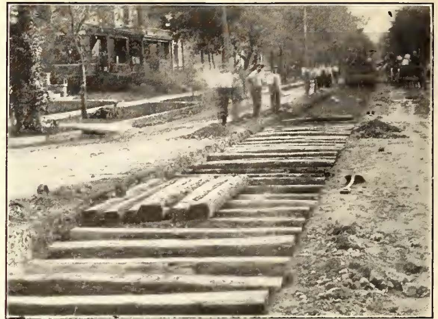
TRACK-TRENCHING MACHINE—VIEW OF INTERVAL BETWEEN TRACK AND EXCAVATING GANGS
