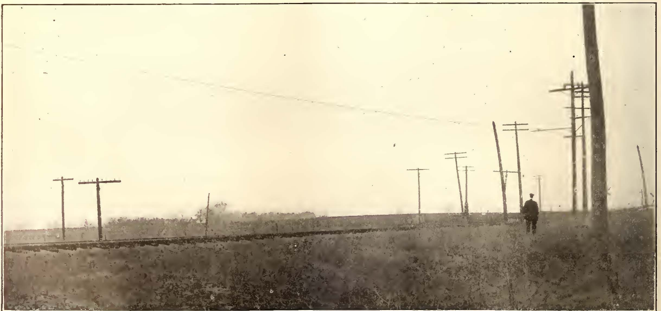
SAFETY TROLLEY HANGER—CUT TROLLEY WIRE HELD BY HANGER
