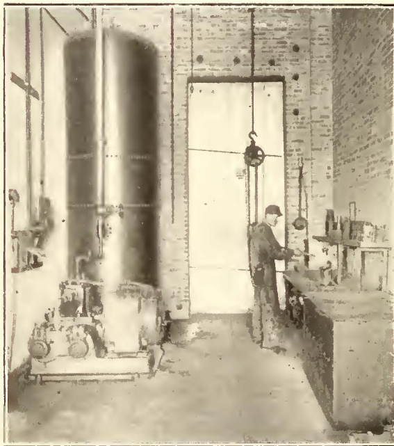
MONROE SHOPS—BABBITTING JOURNAL BRASSES; INTERIOR VIEW OF MACHINE SHOP, SHOWING CRANE
