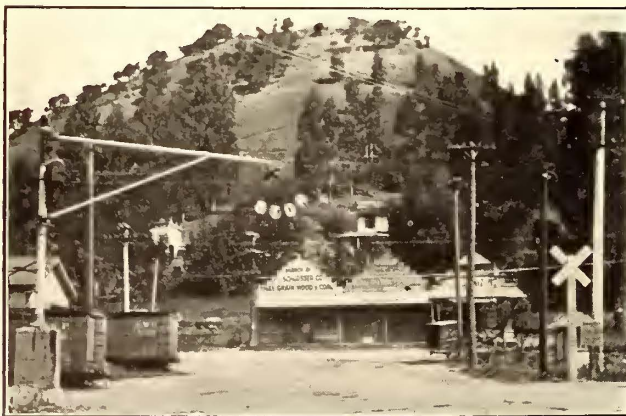
AUTOMATIC WIGWAG CROSSING INSTALLED AT SAN ANSELMO, CAL.
