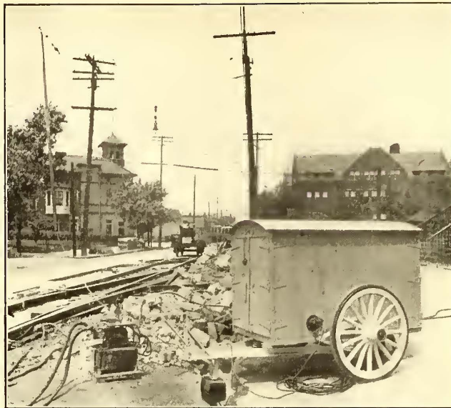
GENERAL VIEW OF CLEVELAND RAIL-BONDING OUTFIT
