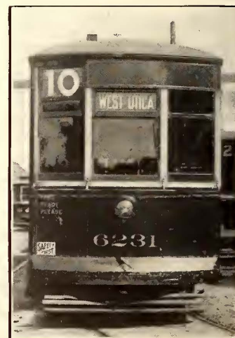
ROUTE SIGNS—VIEW OF INTERNATIONAL RAILWAY CAR, SHOWING LOCATION OF SIDE AND FRONT SIGNS
