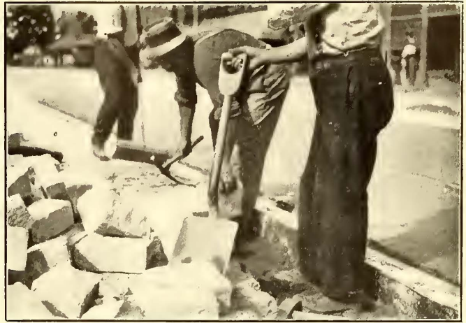
WORCESTER CONSOLIDATED STREET RAILWAY—RELAYING BLOCKS BETWEEN RAIL AND OLD PAVEMENT
