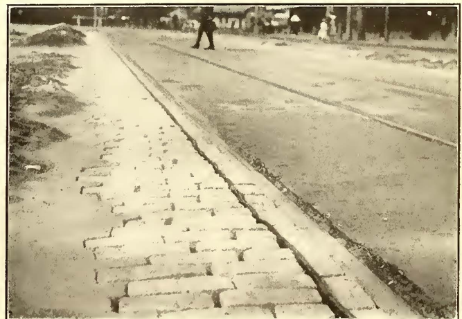
WORCESTER CONSOLIDATED STREET RAILWAY—RELAID PAVEMENT WITH EXPERIMENTAL EXPANSION JOINT
