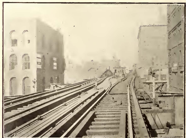
SAFETY ON CHICAGO ELEVATED—VIEW OF DIVERTING TRACK AND SIGNALS AT A CHICAGO RIVER BRIDGE
