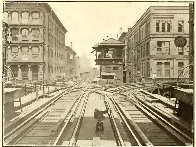
SAFETY ON CHICAGO ELEVATED—VIEW AT JUNCTION SHOWING HEAVY EXTRA GUARD RAILS AND FIRST-AID STATION SIGN
