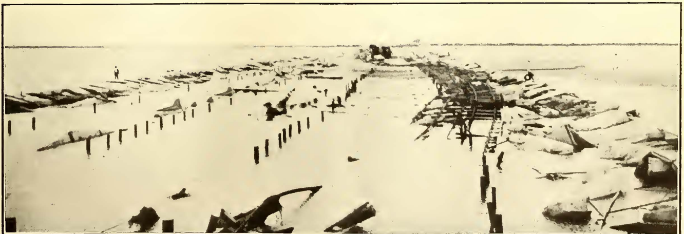
TEXAS HURRICANE—VIEW OF THE GALVESTON CAUSEWAY, SHOWING WRECKED INTERURBAN CAR
