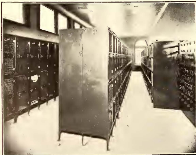
CLEVELAND OPERATING STATIONS—VIEW IN STATION LOCKER ROOM
