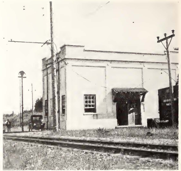
Concrete Substation at Orrville, Oregon Electric Railway
