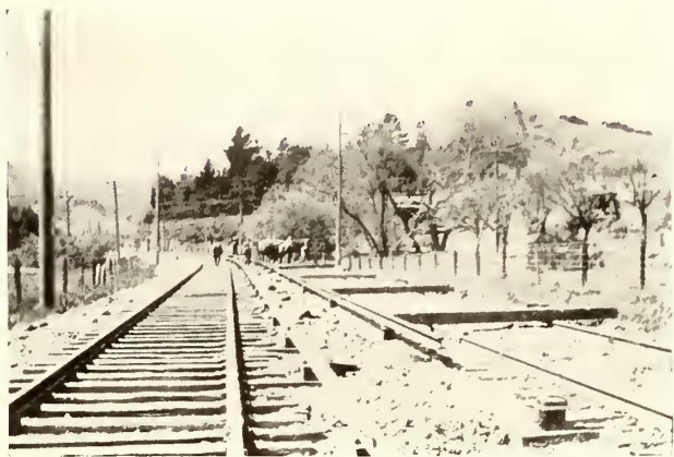
Fifth Step in Moving Live Conductor Rails
