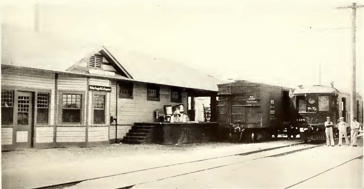
Typical Pacific Electric Local Station at Gardena, on the Redondo Line, with One Freight Car and One Express Car
