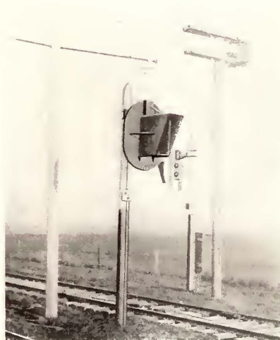
Side View of Light Signal
