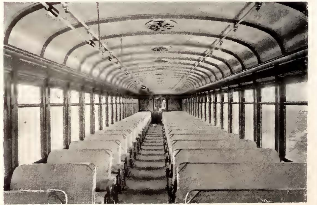
Interior View of Southern Pacific Electric Car
