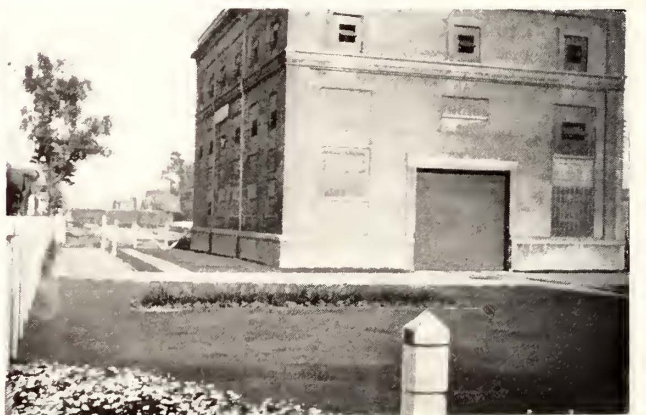
West Oakland Substation and Flower Garden
