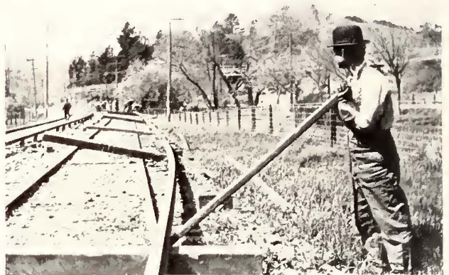
Second Step in Moving Live Conductor Rails
