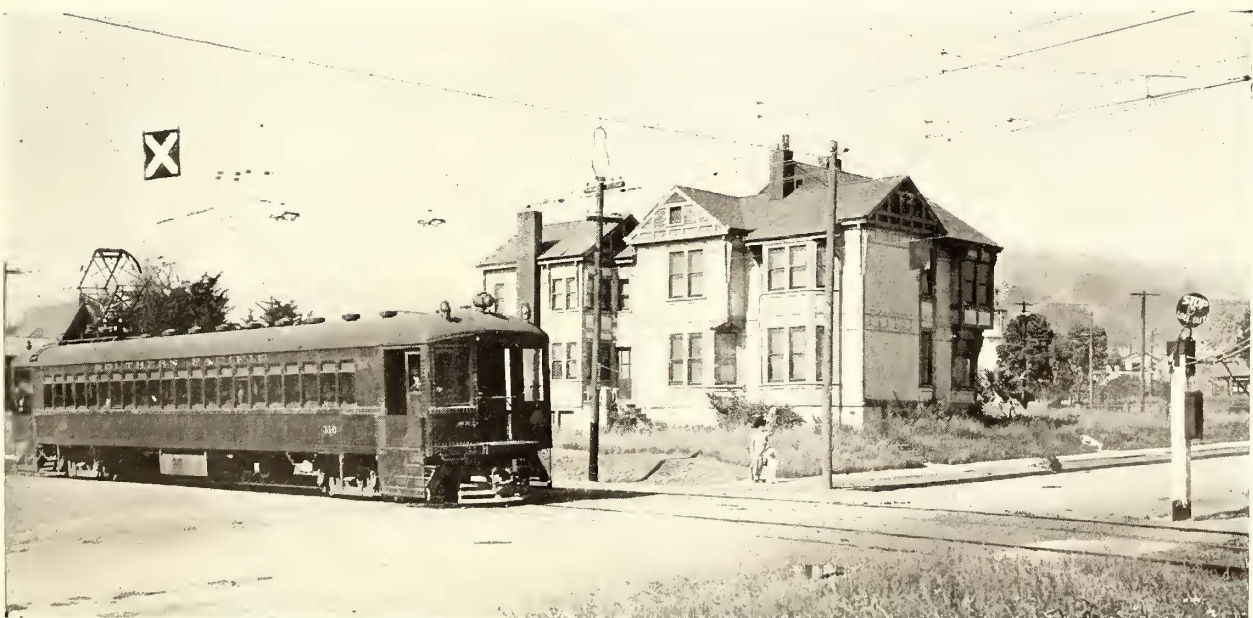
Automatic Wigwag Danger Signal at Berkeley
