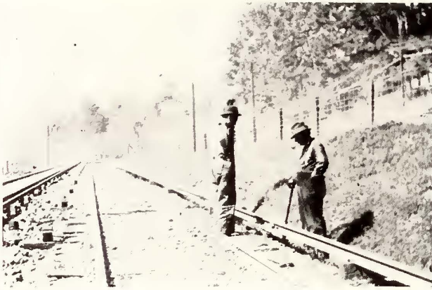
First Step in Moving Live Conductor Rails
