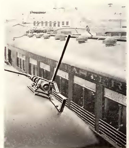
Automatic Train Stop in Key Route
