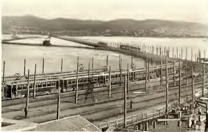
Pier Terminal Yard, Showing New Construction with 2-Mile Fill
