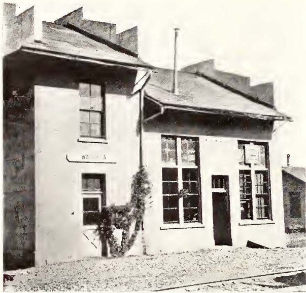
Substation and Agent's Office Combined, Oregon Electric Railway
