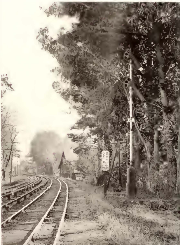
Twelve-Year Old A.C. Track Circuit Signals at Ross
