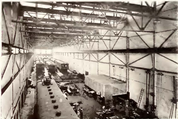
Car Repair Room, Southern Pacific Shops, Alameda Point
