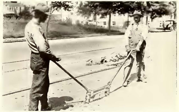
Rail Planer on Grand Avenue, Oakland
