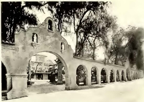
Glenwood Inn, Riverside
