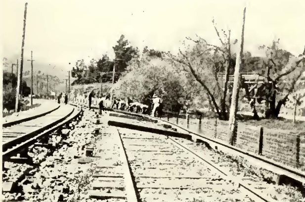
Third Step in Moving Live Conductor Rails
