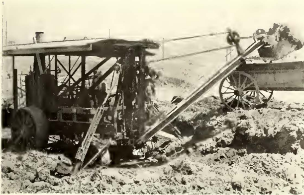
Traction Excavators Used on Trench Excavation on Park Street, Alameda
