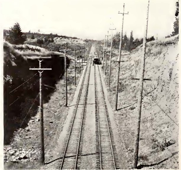
Double-Track Tangent, Oregon Electric Railway, Between Portland and Garden Homes
