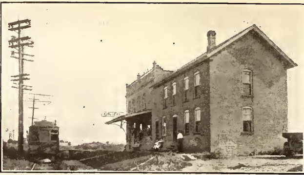
AUTOMATIC SUBSTATIONS—EXTERIOR OF UNION SUBSTATION
