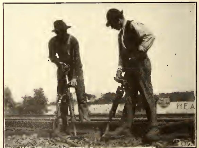
PNEUMATIC TIE TAMPERS IN OPERATION
