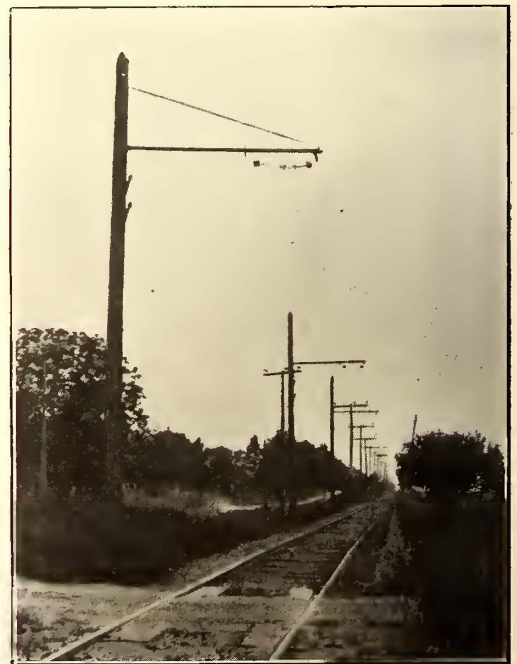
5000-VOLT D.C. EQUIPMENT—CARS AND OVERHEAD CONSTRUCTION ON GRASS LAKE (MICH.) LINE
