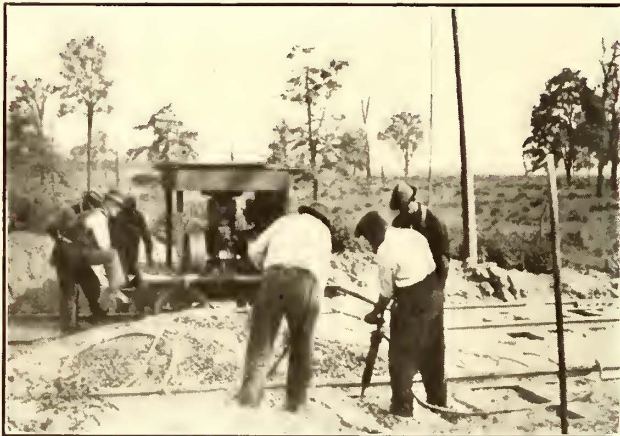
TAMPING OUTFIT ON CLEVELAND RAILWAYS
