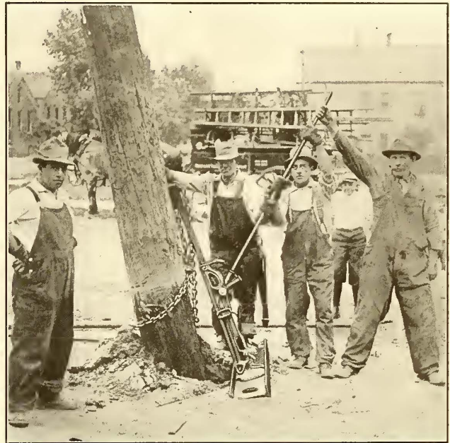
SINGLE-ACTING, 15-TON POLE JACK WITH 24-IN. LIFT
