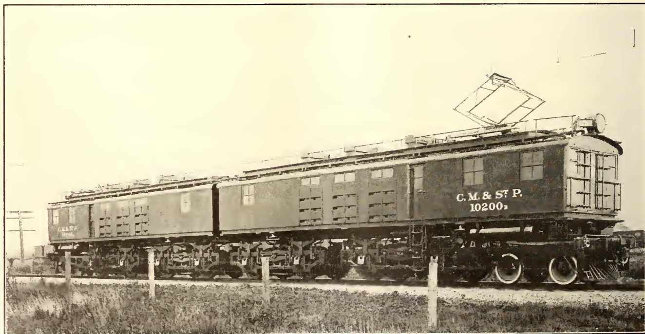
CHICAGO, MILWAUKEE & ST. PAUL ELECTRIFICATION—282-TON, 3000-VOLT DIRECT-CURRENT LOCOMOTIVE IN EXPERIMENTAL OPERATION ON TEST TRACK
