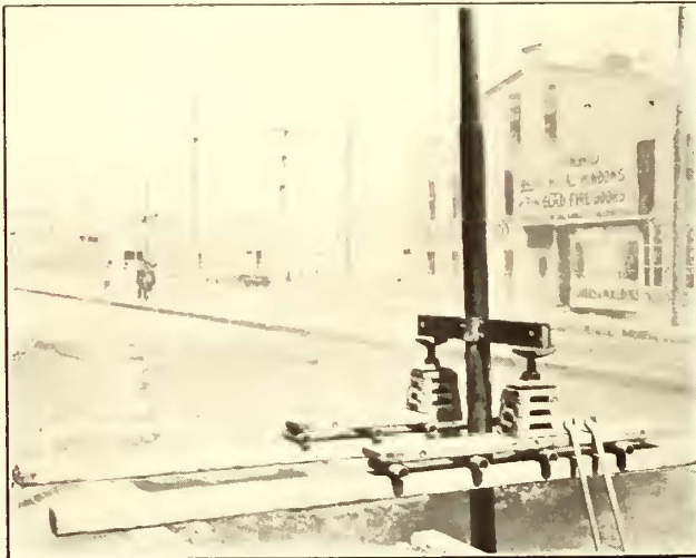
POLE-MOVING APPLIANCE USED IN SAN FRANCISCO
