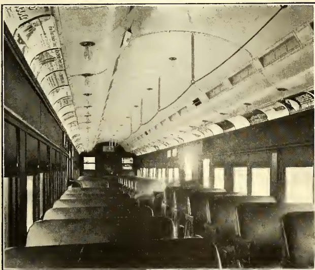
WESTCHESTER LIGHTING—ORIGINAL ARRANGEMENT WITH SMALL LAMPS UNDER DECKS AT EACH SIDE AND EMERGENCY LIGHTS IN THE CENTER
