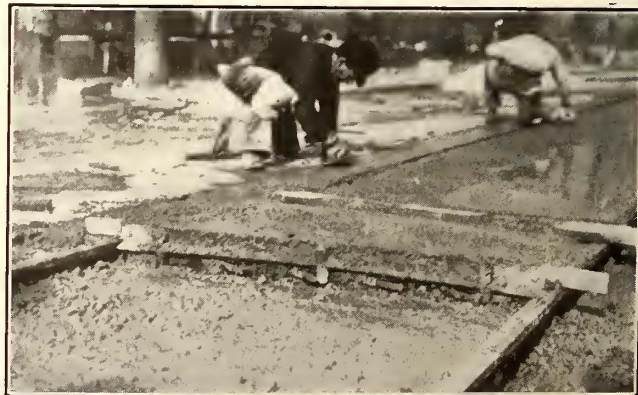
CONCRETE PAVEMENT—FLOATING SURFACE TO FINISH AFTER STRIKING OFF WITH TEMPLATE
