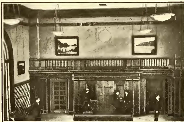
INTERIOR OF PASSENGER STATION AT EUGENE
