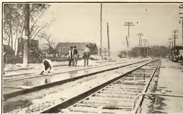
CONCRETE PAVEMENT—COMPLETED STRETCH OF CONCRETED TRACK
