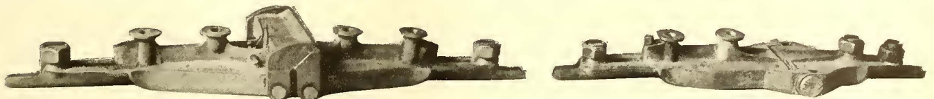
POSITION OF FROGS WITH BRIDGE CLOSED, SHOWING CONTACT FROGS TOGETHER AND HINGED FROG STRAIGHT
