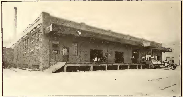
CLEVELAND REPAIR SHOPS—VIEW OF FRONT OF STOREROOM BUILDING
