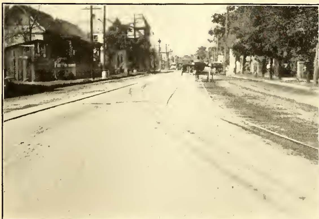
HOUSTON PAVEMENT—BRICK ON MORTAR WITH GROUT FILLER LAID JANUARY, 1912, 7-IN. T-RAIL
