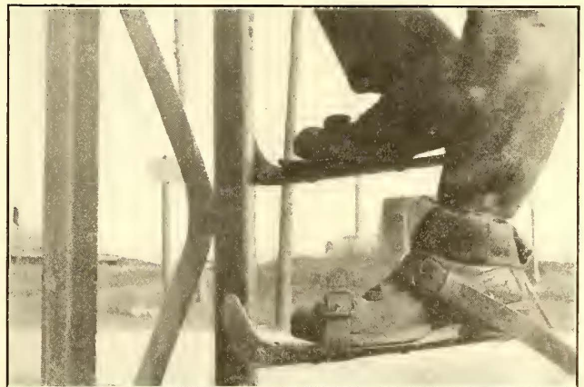
STEEL POLE CLIMBERS IN ACTUAL OPERATION
