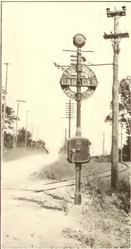
HIGHWAY CROSSING SIGNAL—SIGNAL INSTALLED ON CONCRETE FOUNDATION; STOPPING CONTACTOR; MOTORMEN'S INDICATOR
