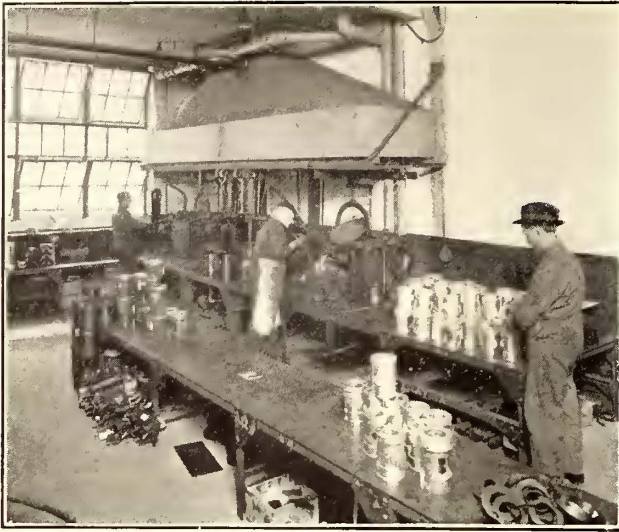
CLEVELAND REPAIR SHOPS—VIEW OF BABBITTING EQUIPMENT
