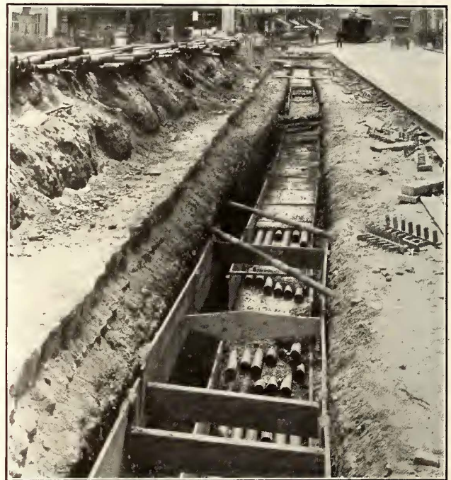
FIBER CONDUIT FOR RAILWAY FEEDERS AND OTHER CIRCUITS AT WORCESTER, MASS.
