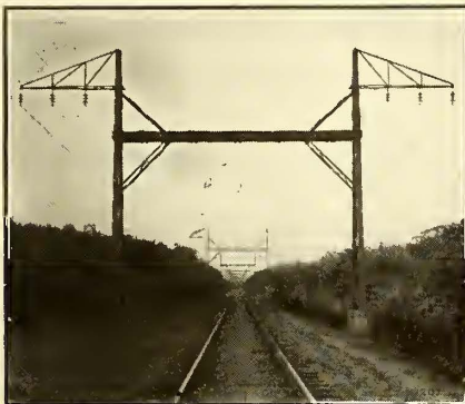
Track Spans, Panama
